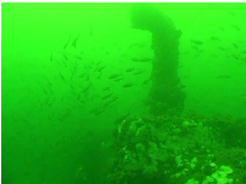
View of one of the brine discharge diffusers
